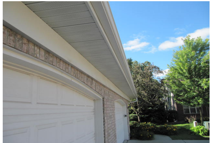
Soffits at garage door.
