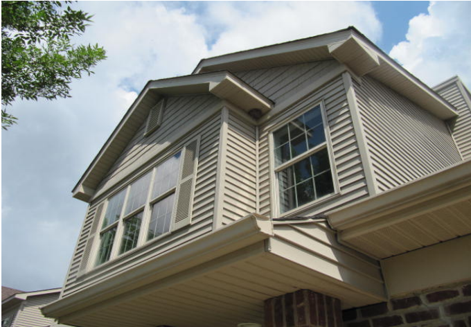
Soffits and fascia at gables and front entrance,
