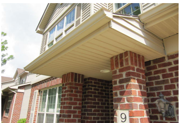
Front entrance soffit.
