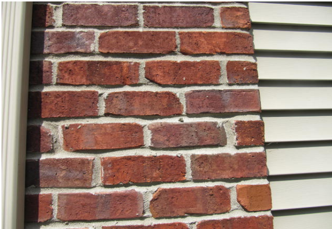
Masonry, typical condition.
