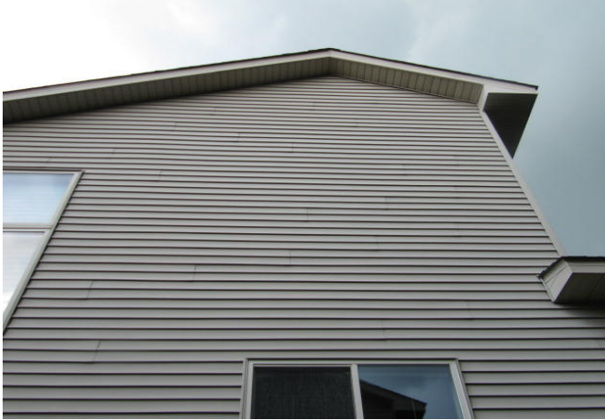
Vinyl siding overview.
