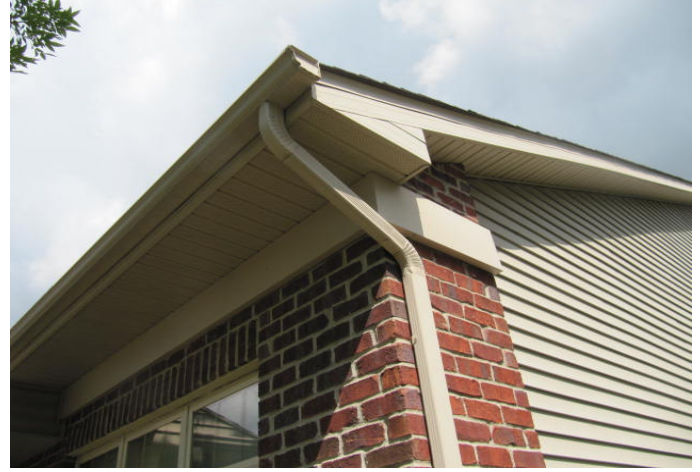
Gutter and downspout at roof line.
