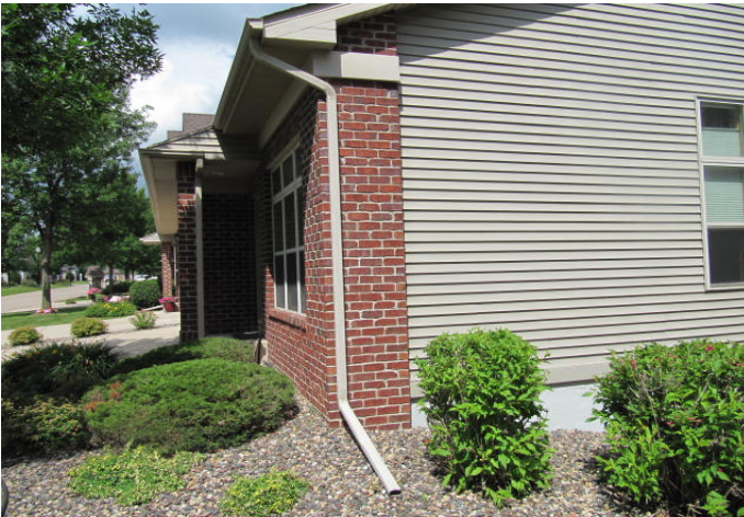
Downspout at corner of building.
