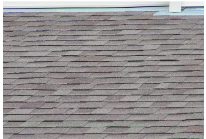
Shingles, good condition.
