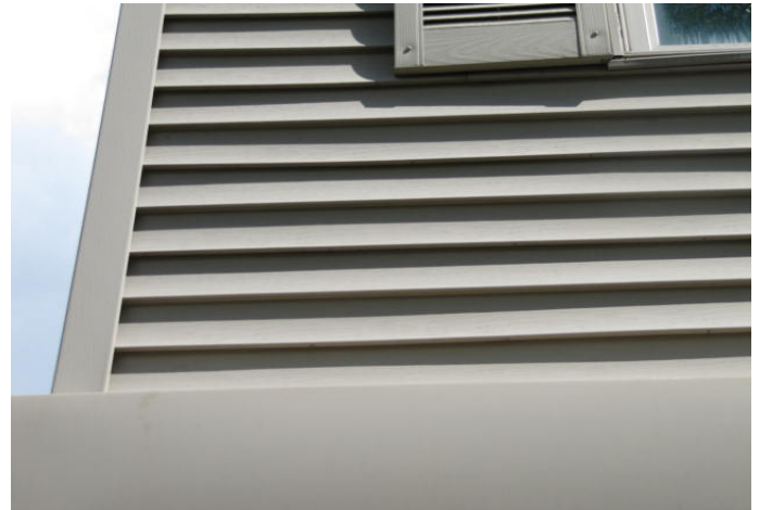
Siding detail, good condition.
