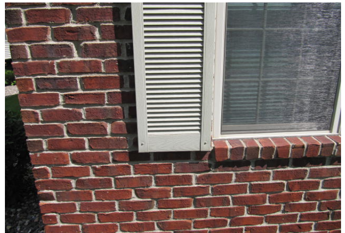
Shutter in good condition.
