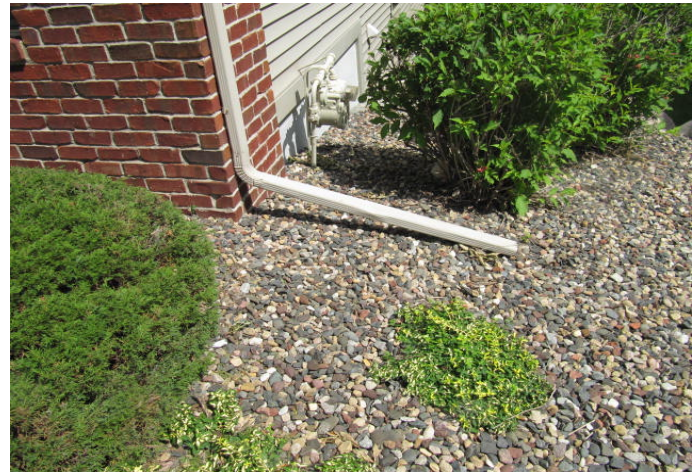
Downspout at grade,
