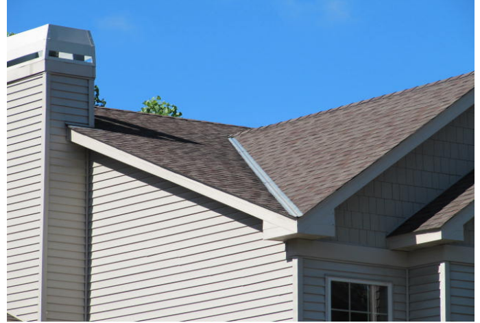
Shingles at roof valley.
