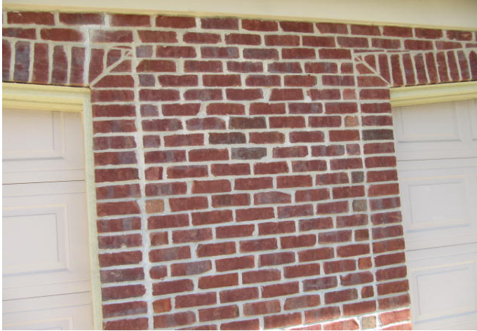
Typical masonry at front of building.
