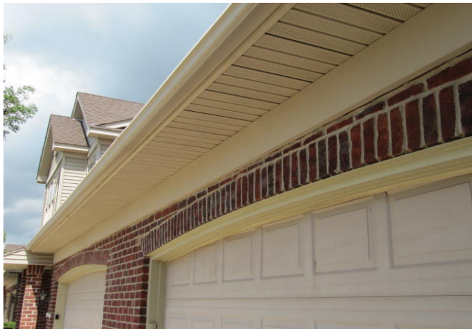
Soffits in good condition.
