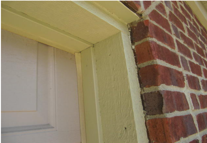
Wood trim paint, good condition.
