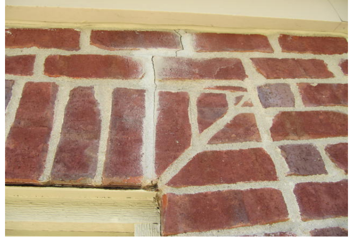
Masonry above garage door.
