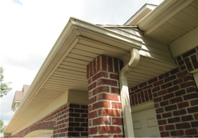
Front of building with gutter and downspouts.
