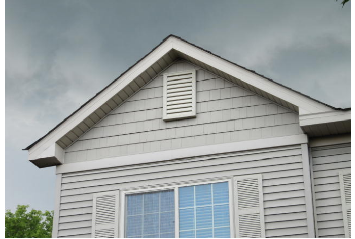
Vinyl siding at gable.
