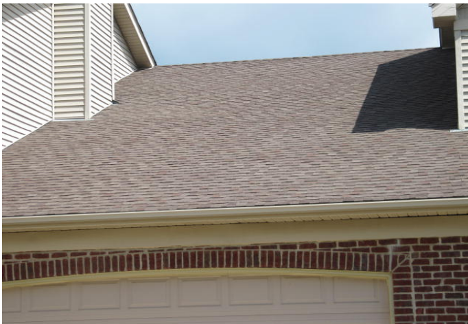
Roof, typical condition.
