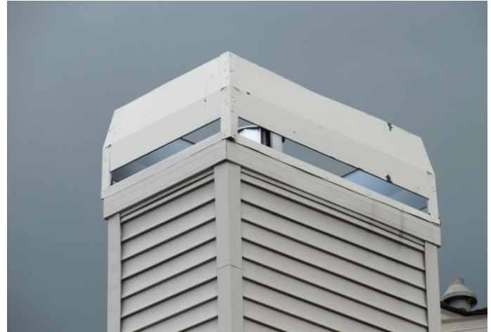
Chimney cap behind cap trim.
