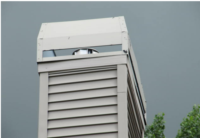
Chimney cap, typical.
