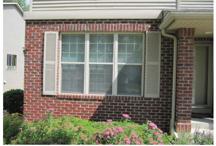
Shutters at first floor window.
